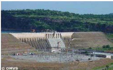
Figure 4: Manantali Dam on Senegal river
