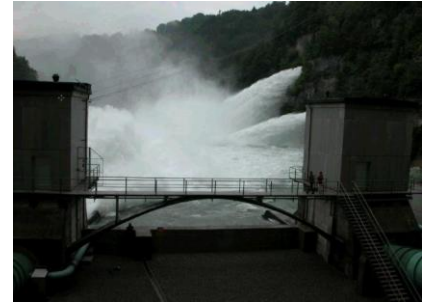
Figure 2: reserve storage for flood protection
