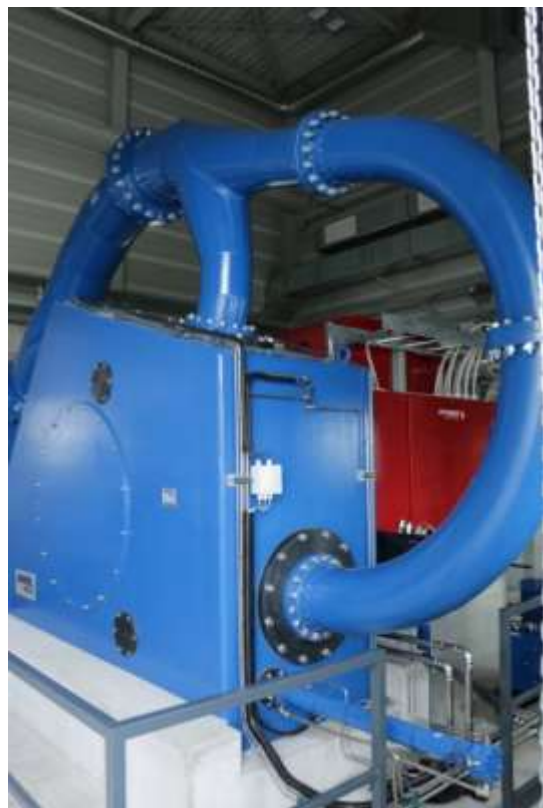
Morgental, St. Gallen, Switzerland 190m, 850 l/s, 1,300 kW
