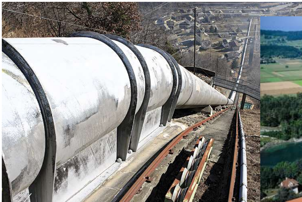
KW Campocologno, Switzerland 50 MW, 13m 3 /s
