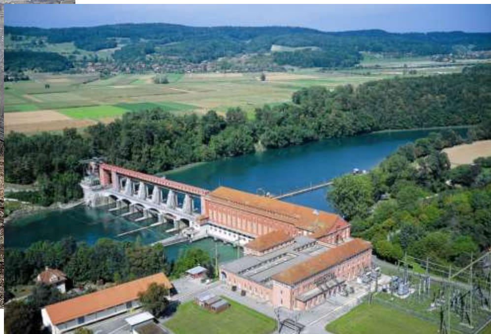
KW Niedergösgen, Switzerland 49 MW, 380 m 3 /s
